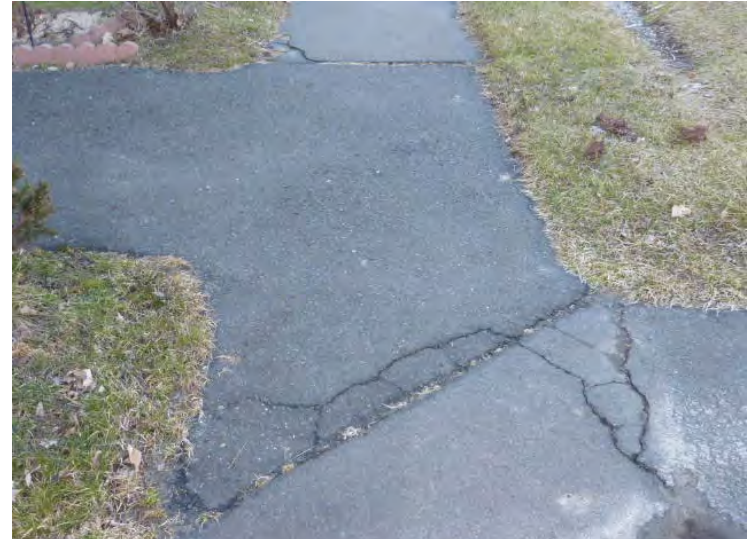
Typical asphalt walk paving has field and edge failures due to inadequate sub-base.
