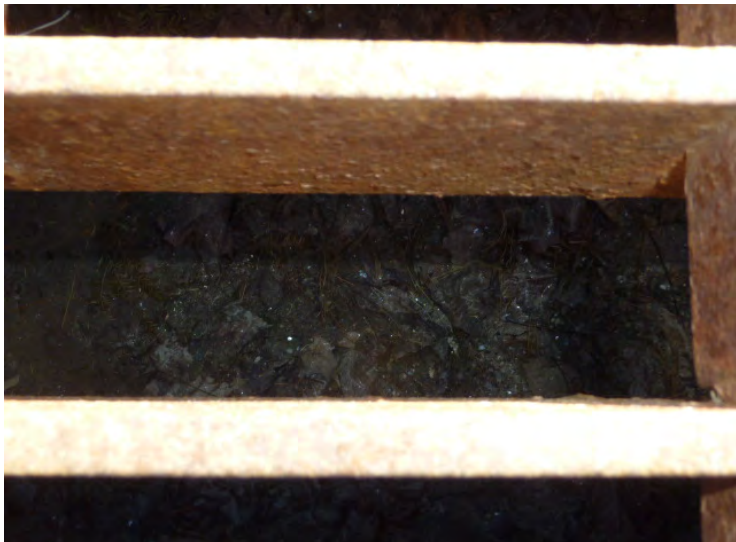
Catch basins on storm water drainage system are full of debris and shown to be cleaned in Year 1.
