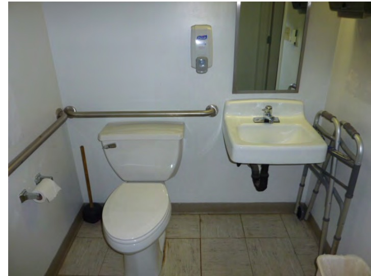
Spacing of toilet and sink in Community Room do not comply with ADA spacing requirements.
