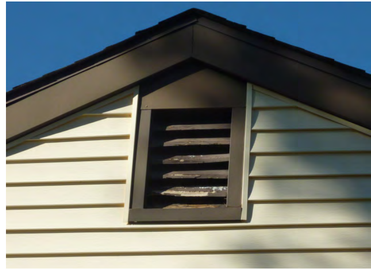
Wood attic ventilation grilles should be repaired and painted site wide by maintenance.
