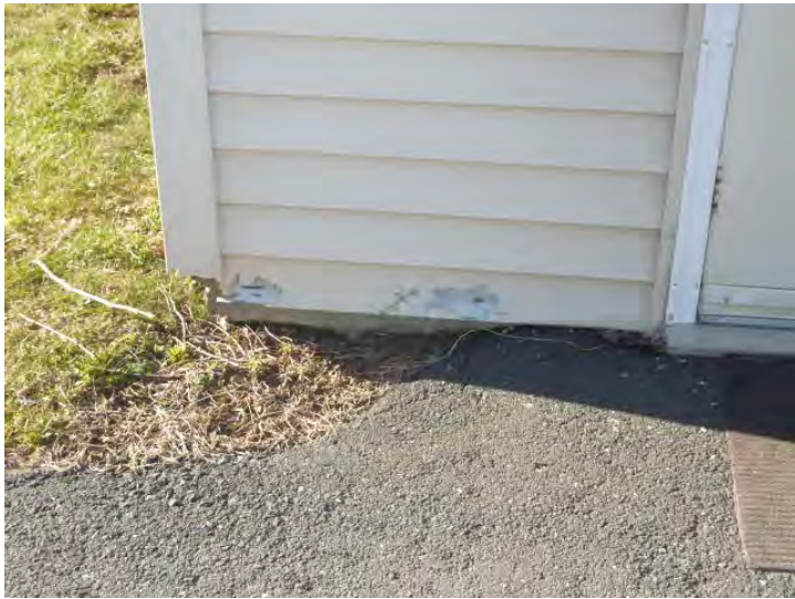
Typical vinyl siding damage.
