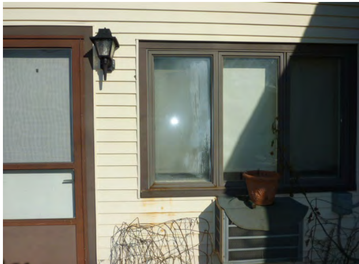
Unit and screen doors have failed finishes and are well worn. Typical condensation inside the insulating glass due to seal failure.
