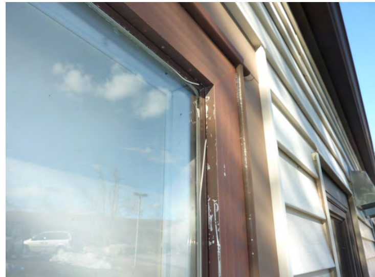
Typical gasket failure at storm doors.
